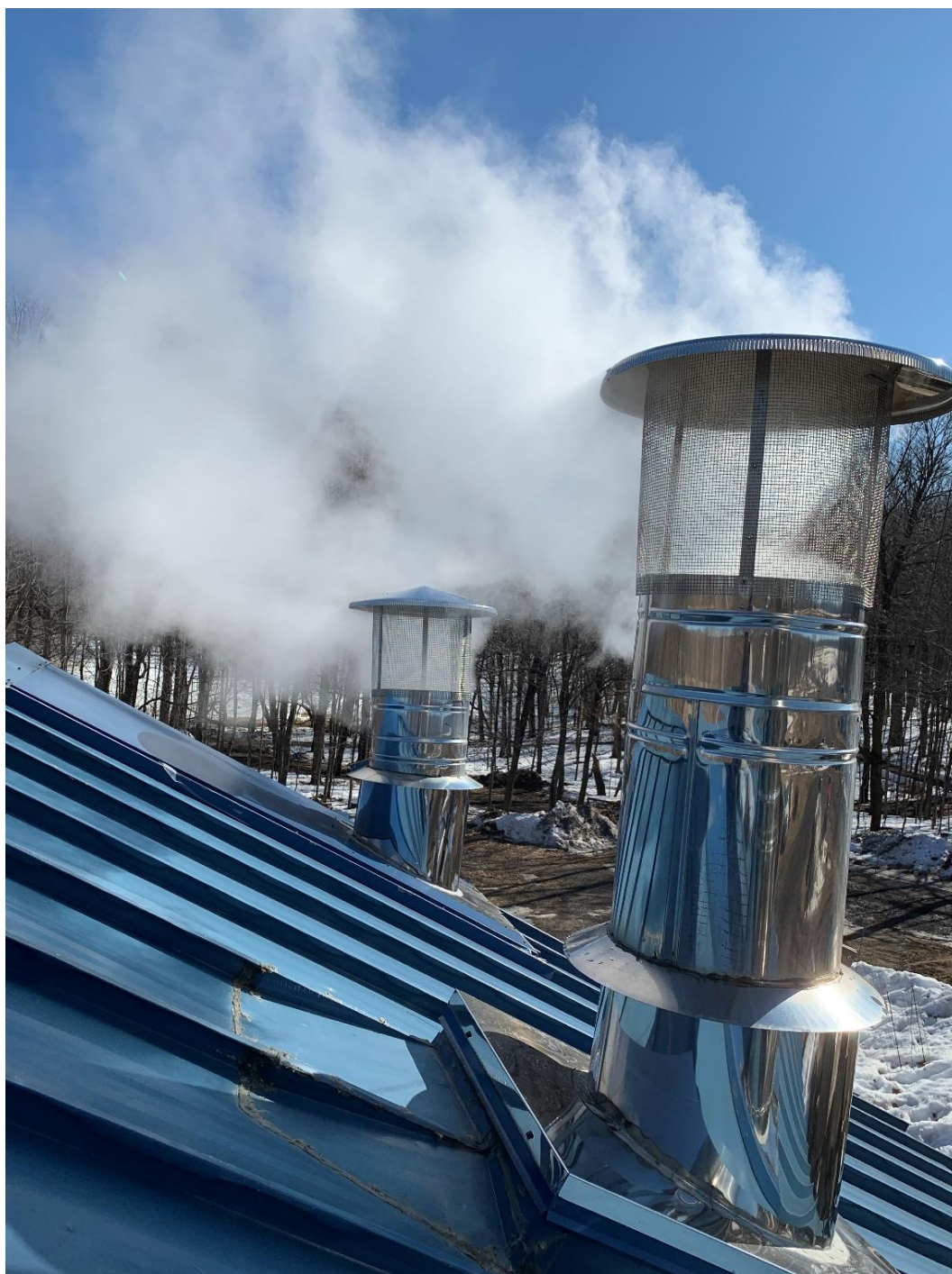
Figure 24. Roof-top view of the steam stacks of Big Burnie.
