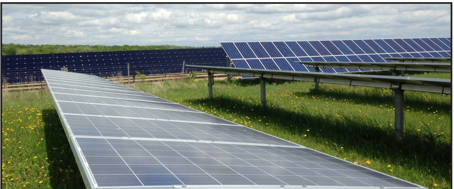
Saint John's Abbey Solar Farm provides many opportunities for research with three different installations of solar technology. The first four-acre installation (pictured in foreground) installed in 2009 automatically tracks the sun throughout the day. A second installation of non-tracking panels was installed in 2014 (top right) around the perimeter of the original installation. And in January 2017 the Orion Solar Garden added an additional 23 acres of solar technology (darker panels pictured in back). KYLE RAUCH.
