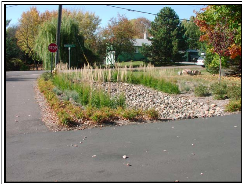
Figure 2 – Illustration of a roadside rainwater garden
