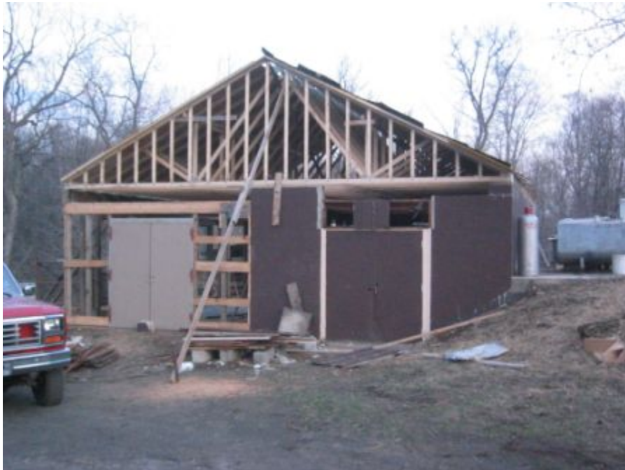
Fig 4. Sugar house addition (photo by Br. W. Kieffer, OSB)
