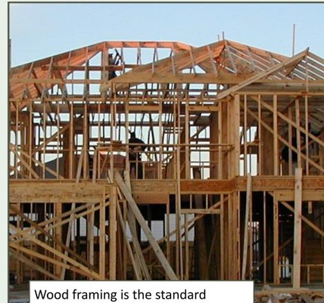
Wood framing is the standard method of home construction in the U.S. usually consisting of 2"x4" or 2"x6" dimensional lumber and fiberglass insulation. While it is a quick and inexpensive way to build, it lacks in energy efficiency.
