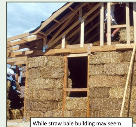
While straw bale building may seem primitive, it is actually highly efficient and the materials can often be sourced locally and inexpensively. Though not shown here, it is generally covered with plaster once construction is complete, to seal out moisture and reinforce the structure.
