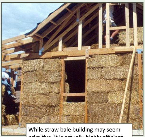
primitive, it is actually highly efficient and the materials can often be sourced locally and inexpensively. Though not shown here, it is generally covered with plaster once construction is complete, to seal out moisture and reinforce the structure.
