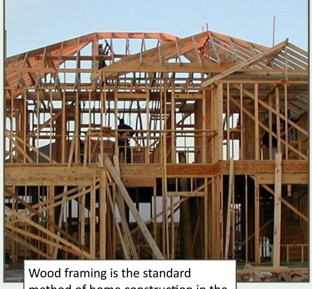
method of home construction in the U.S. usually consisting of 2"x4" or 2"x6" dimensional lumber and fiberglass insulation. While it is a quick and inexpensive way to build, it lacks in energy efficiency. Photo: http://en.wikipedia.org/wiki/File:Wood-framed\_house.jpg
