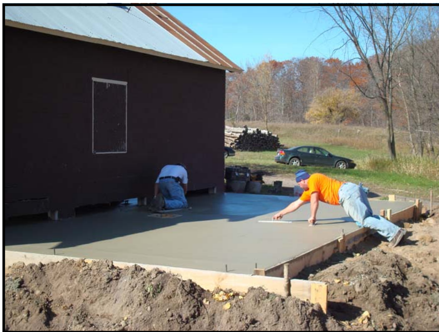
Workers lay concrete for the expansion of the maple syrup sugar shack.
