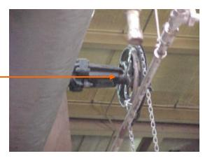
Step 4: Close atomizing steam valve on header. Apply locking mechanism (such as a saftee donut) and secure with padlock. Apply tag.
