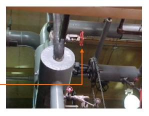
Step 5: Close two (2) gas valves. Apply locking mechanism (such as ball valve lockouts) and secure with padlocks. Apply tags.
